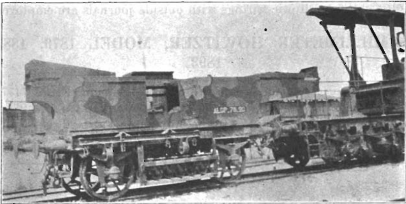
SHUTTLE CAR OR TRANSBORDEUR FOR DELIVERING AMMUNITION TO SLIDING MOUNTS FROM DUMP OR CAR IN REAR.
