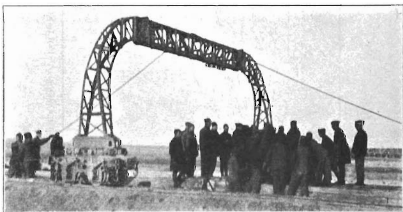
SETTING UP ROLLING BRIDGE.
