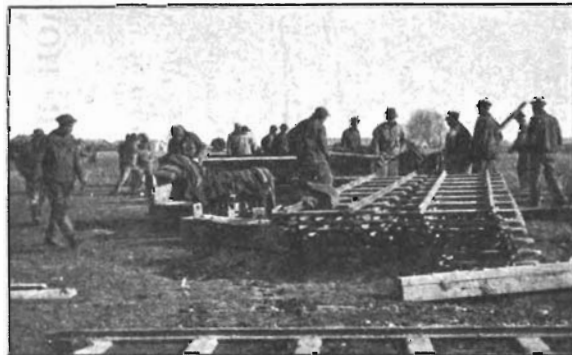
SCENES INCIDENT TO INSTALLING EMPLACEMENT FOR 340 GUN RAILWAY MOUNT.
